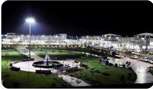
External Lighting - APIGC
